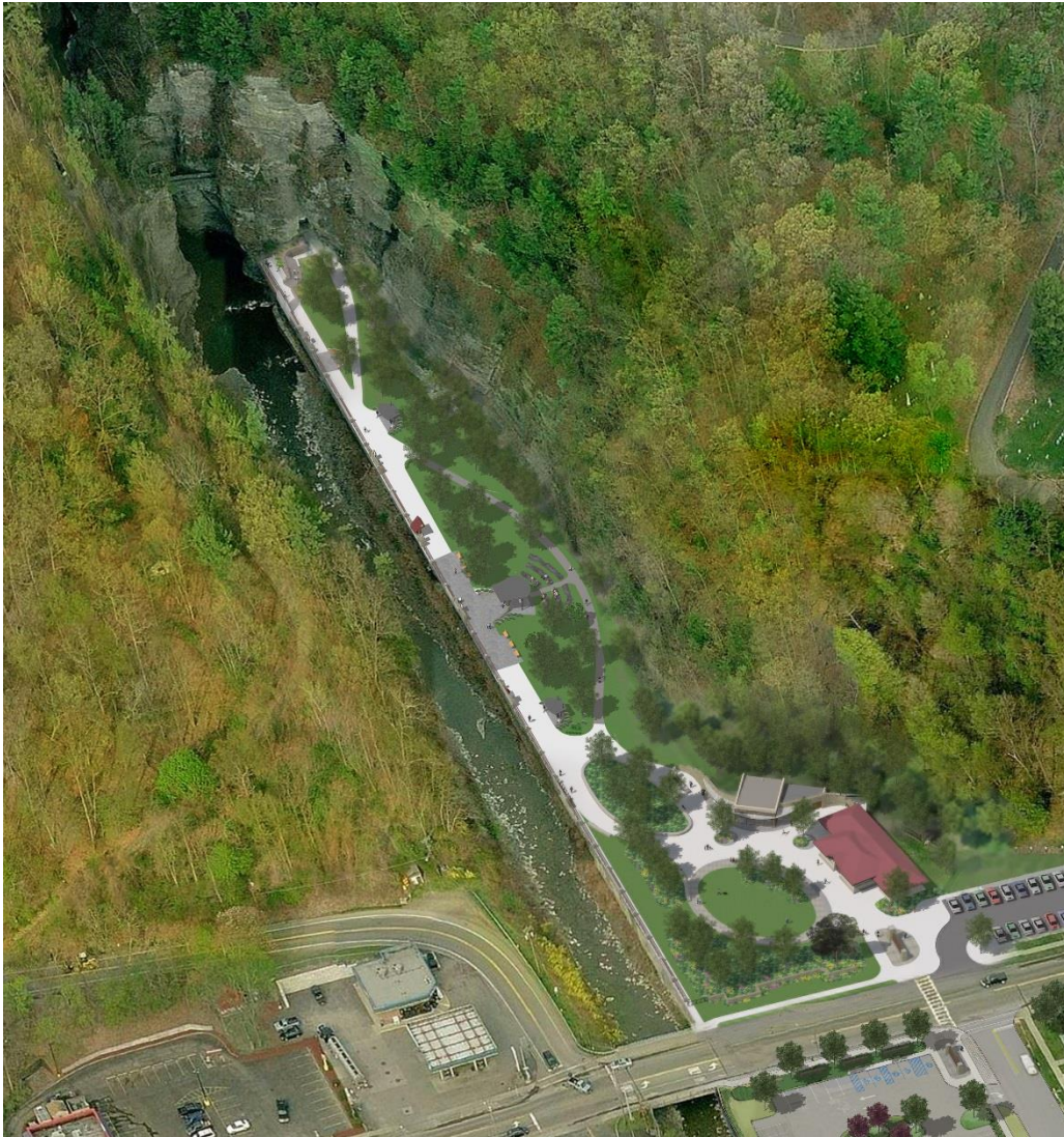
Birdseye view of the renovated entrance and addition of green space along the Creek walk to the entrance of the Gorge Trail
